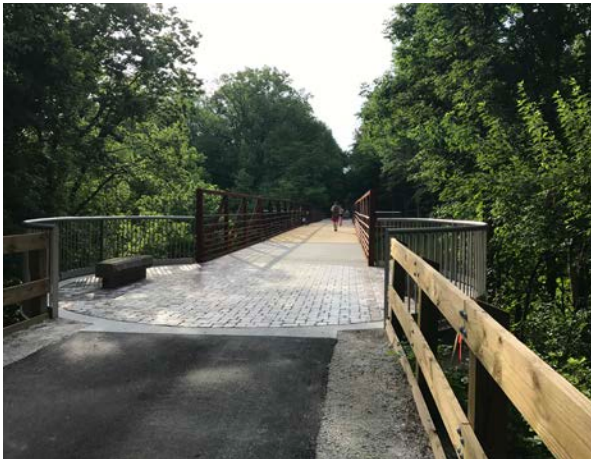
135-foot long weathering steel truss bridge over White Lick Creek on the B&O Trail in Hendricks County
