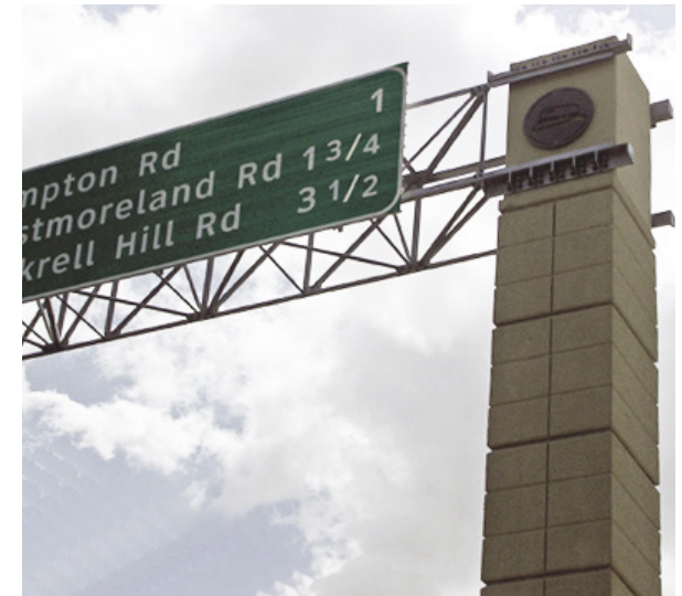
Example of similar interstate sign structure support
