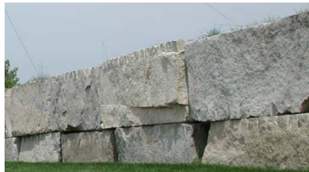
5'x8' Indiana limestone quarry blocks
