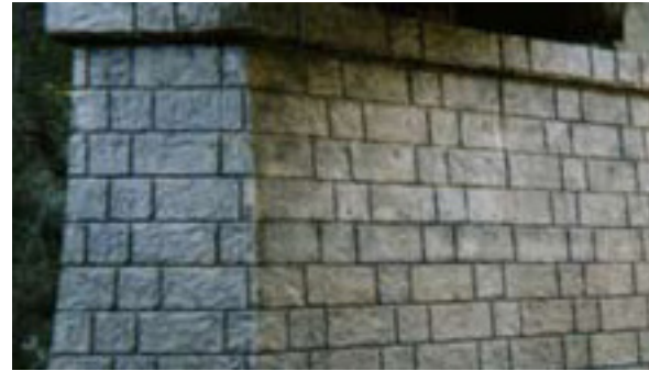
Form liner variant of Limestone coursing
