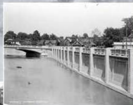
Fall Creek Flooding A flood devastates Indianapolis in 1913 (left), killing 200 people. Kessler designed concrete floodwalls (above) and earthen levees in the City Beautiful style to control water levels.
