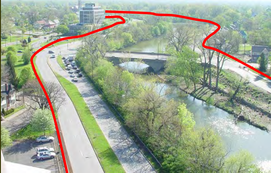
View looking northwest to Delaware Street Bridge
