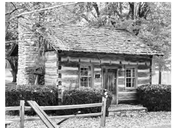
01077 The Samuel Schwartz House, constructed in 1837, is a single-pen log building.
