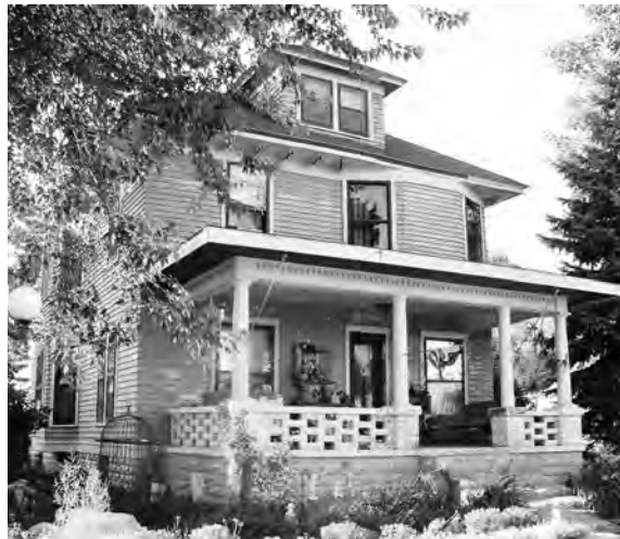
01067 This American foursquare has a high level of historic integrity. Note the use of ornamental concrete block on the porch.
