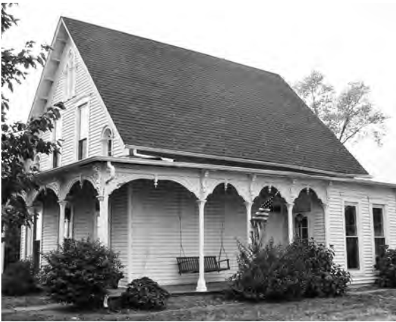
00025 The Horace Solomon House is an outstanding example of a Gothic Revival home that retains many interesting details.
