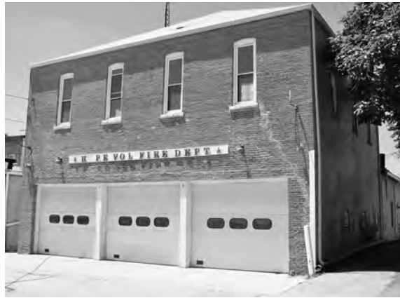
01207 Lodge Hall is an example of a typical two-part commercial block.
