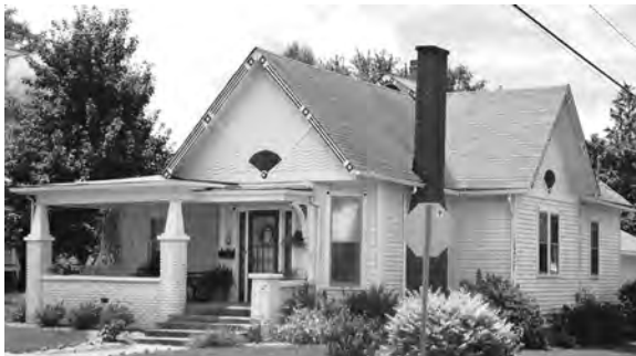
01148 A small cottage with Queen Anne details. The front porch is probably a later addition from the 1920s or 1930s, added to give the house a more Craftsman appearance.
