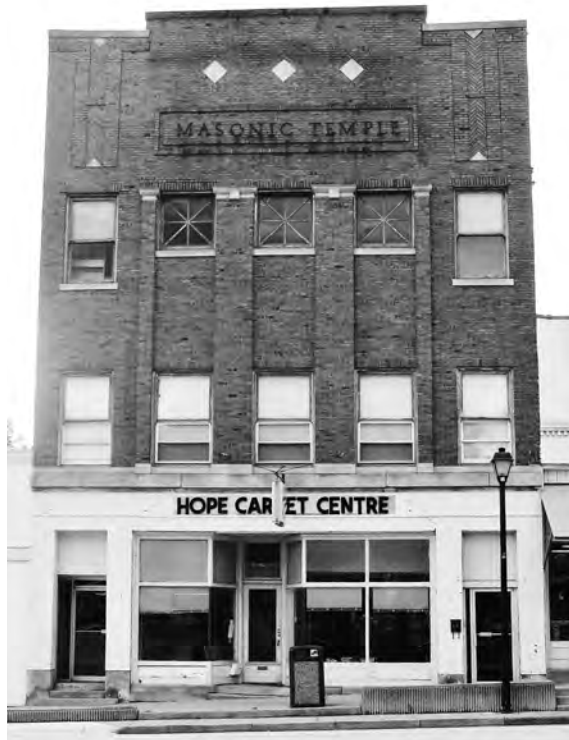
01155 The Masonic Temple features interesting brick corbelling above the third story.
