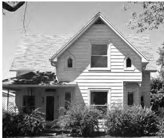
01001 This gabled-ell house from c.1890 has Queen Anne details, such as the use of various window shapes.
