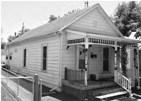
01257 An example of the shotgun form. This house also features porch details that resemble the Queen Anne style.
