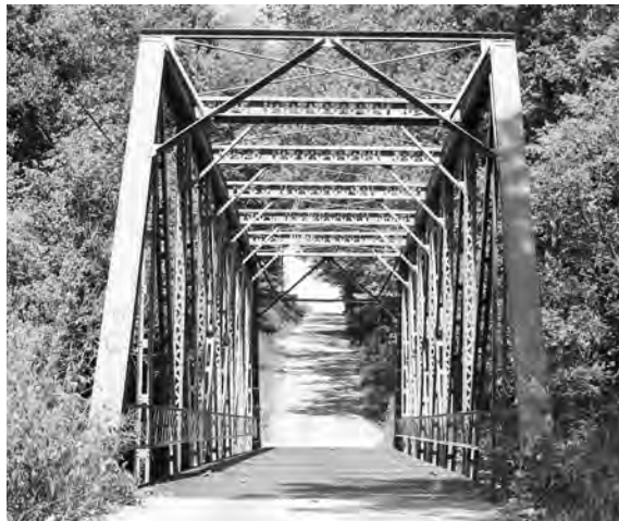
00028 The riveted pratts used on County Bridge No. 47 are rare in Indiana.
