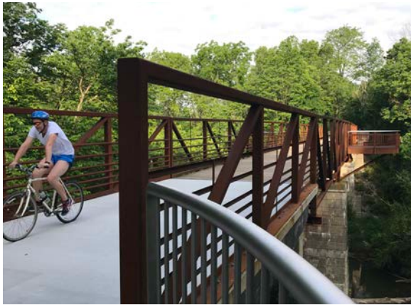
White Lick Creek Trail Bridge
